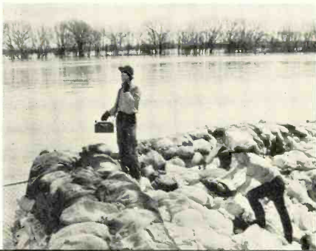
A patrolman, equipped with a two-way radio, reports on the condition of the dikes which were thrown up around the North Omaha pumping station during flood.
